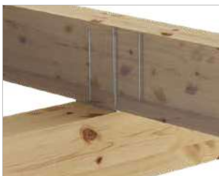
Reinforcement in the point of support
