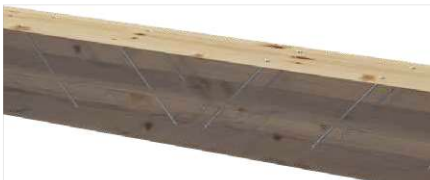
Reinforcement by coupling of beams
