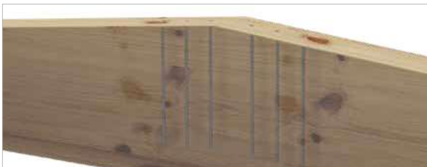
Reinforcement with screws in roof ridge area
