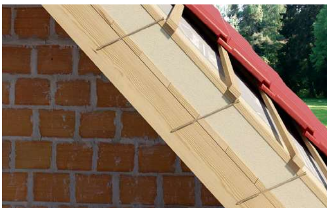
Fixing of rigid insulation
